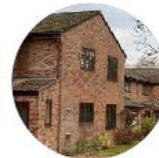
Multi-tonal bricks, corbelling and porches
