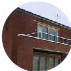
Red brick with timber window and door frames
