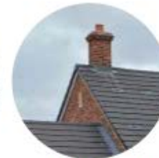
Chimney and slate roofing
