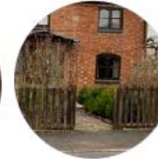
Timber fences and flat arch window
