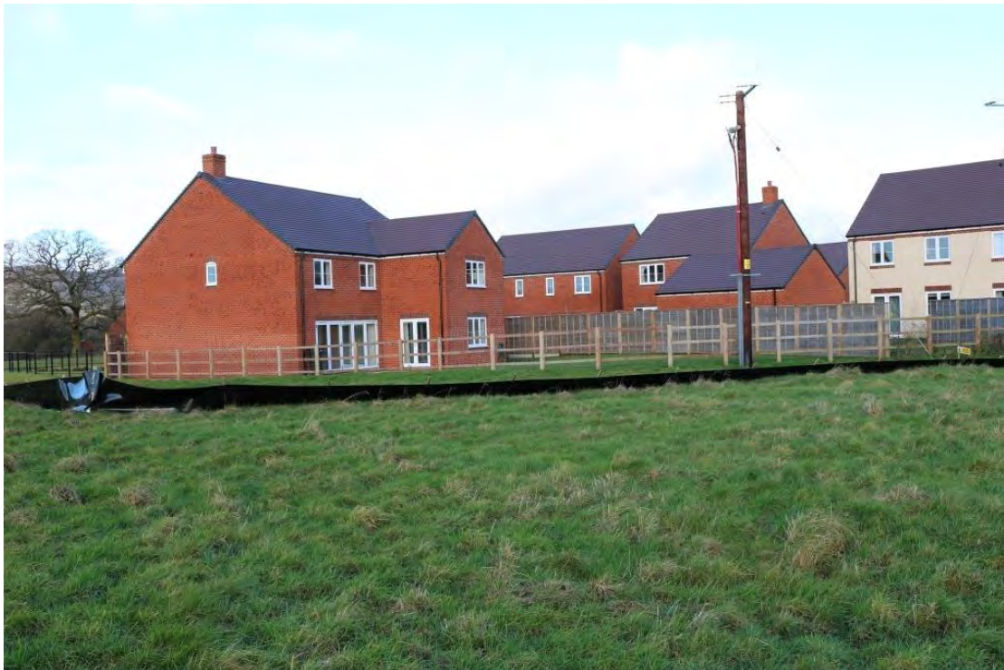
Recently-constructed houses at Lawn Farm, adjacent to Area's northern boundary
