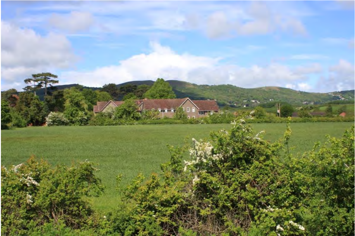
Welland House from south east
