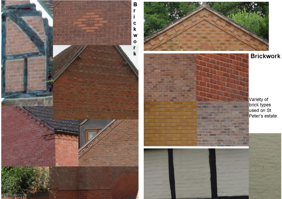
Figure 15: Photographs of Materials and Architectural Details
