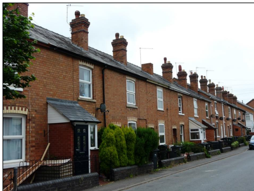
Figure 2 Belmont Road Terraces
