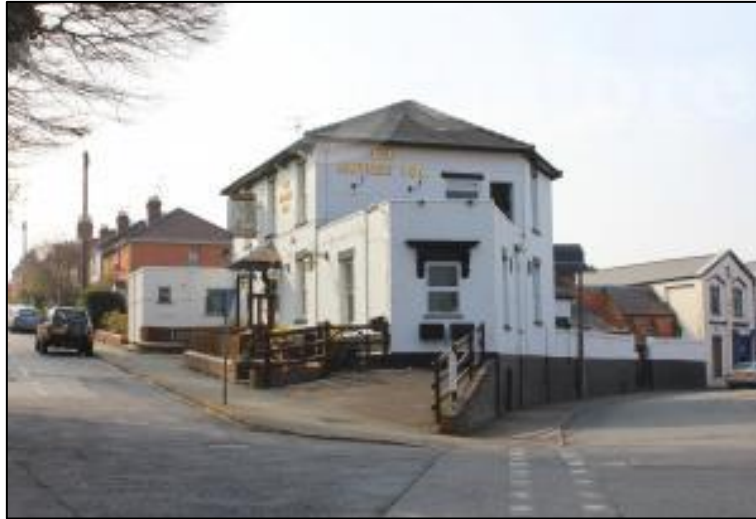
Figure 6 Express Inn showing former Santler building to the right
