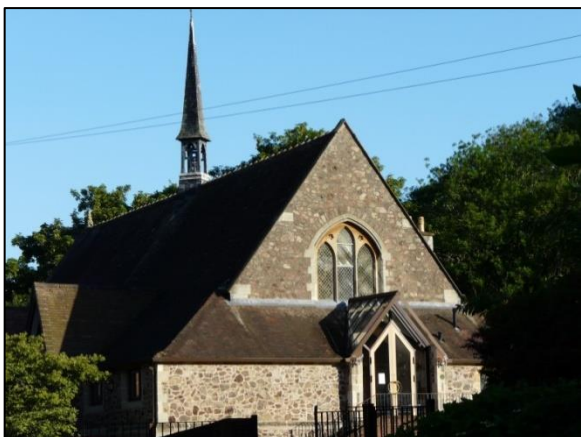
Figure 14 St Joseph's R C Church
