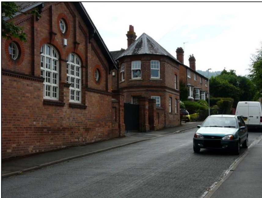
Figure 7 Former Nicholson Organ Factory and unusual pointed bays on adjacent terraced houses
