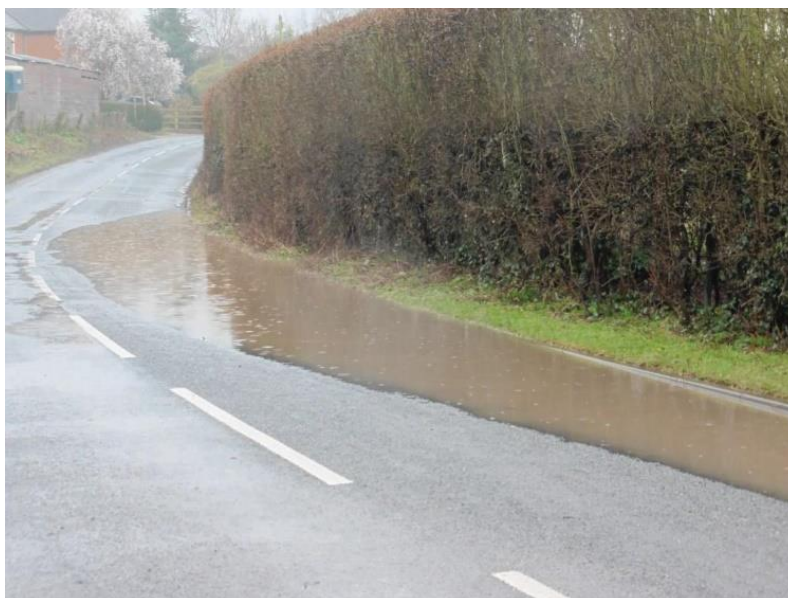
Typical roadside “muddy” flooding
