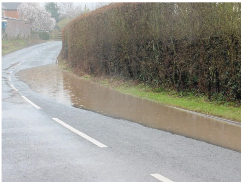
Typical roadside "muddy" flooding
