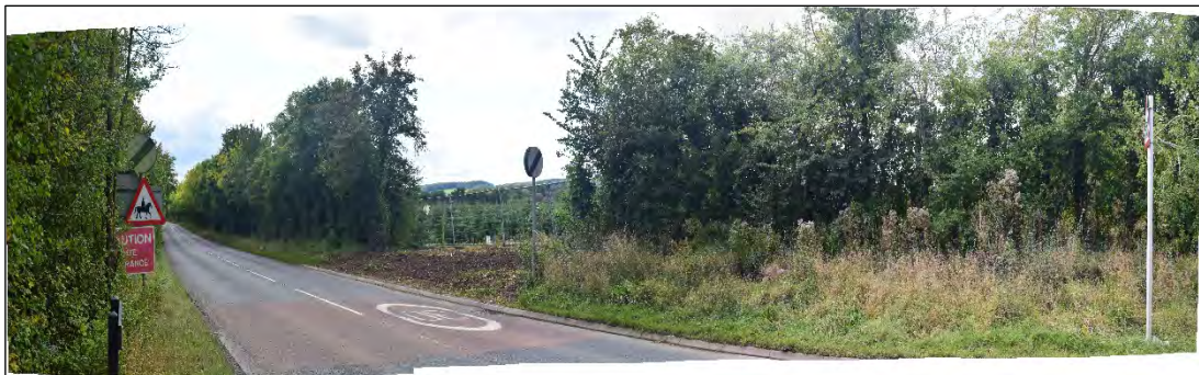
Photo 2 The Site's access from Leigh Sinton Road facing south
