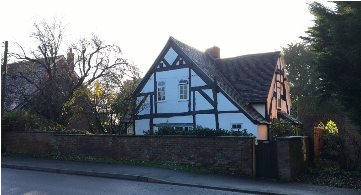
Plate 5: Ahisma Malvern House Cottage, north elevation viewed from the A4103
