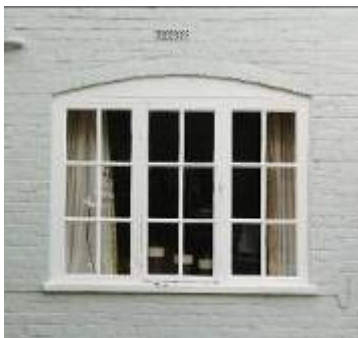
(3 light casement window) (Sash windows with glazing bars)
