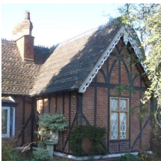
(Bargeboards and decorative roof and ridge tiles)
