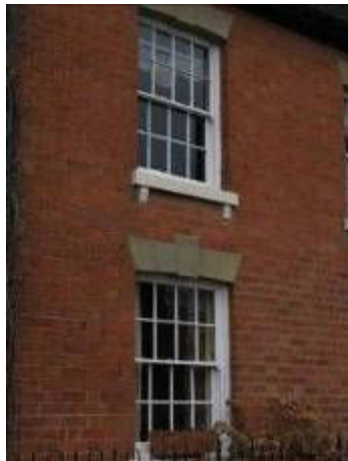
(3 light casement window) (Sash windows with glazing bars)
