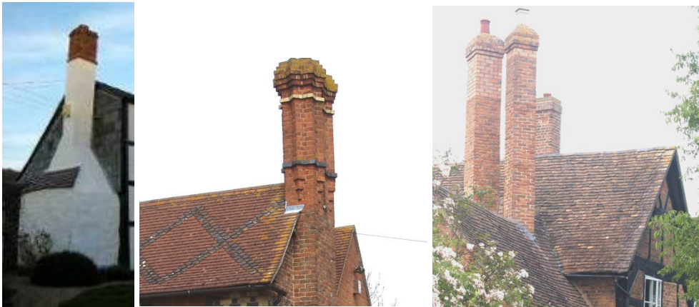
(Examples of traditional chimneys)
