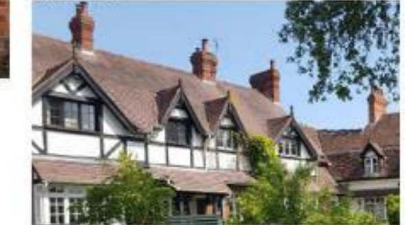
Varied dormer windows
