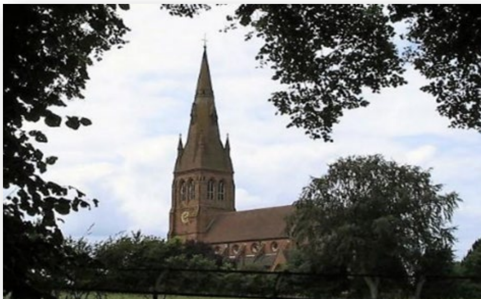
Figure 7: View of Hallow Church from the South
