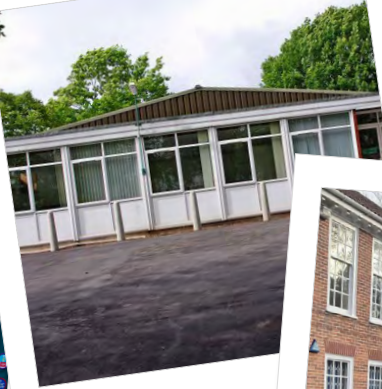
48 village halls and community facilities
