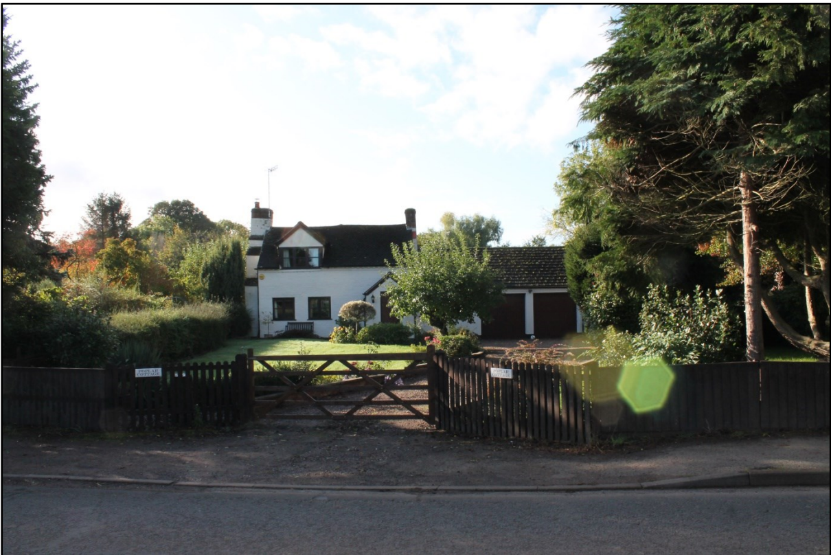
Plate 16: Poplar Cottage, Drake Street
