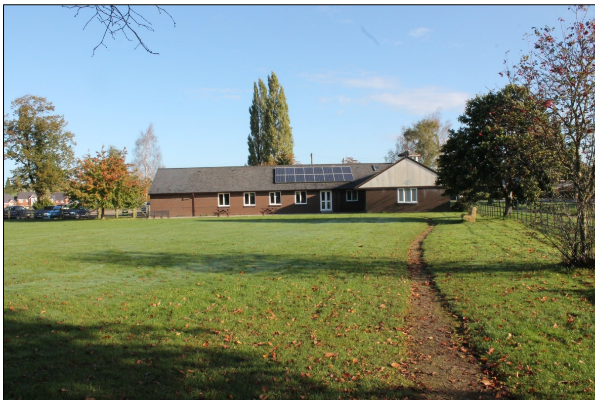
Plate 24: Southern elevation of Parish Hall
