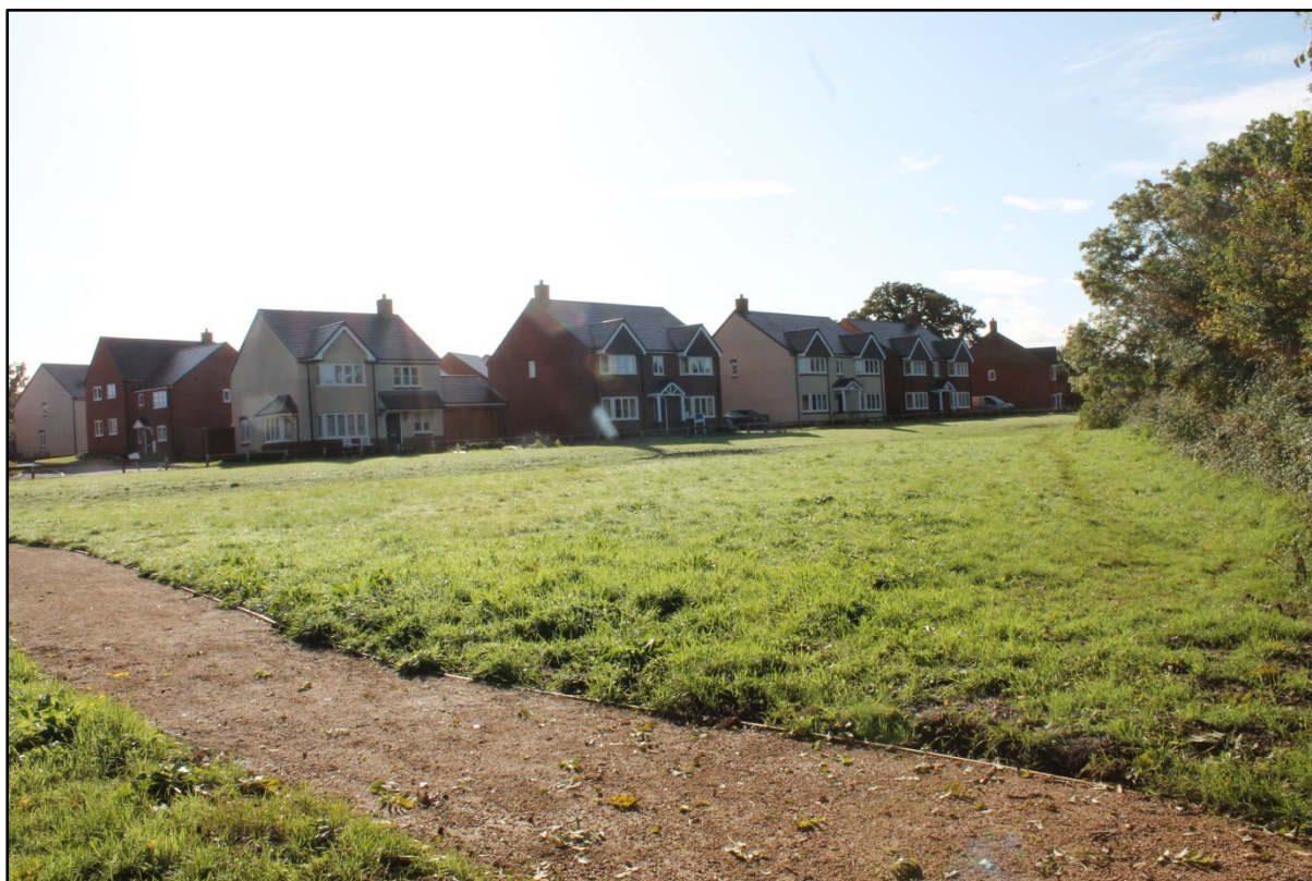
Plate 10: Kingston Close (part of Lawn Farm Phase 2 development)
