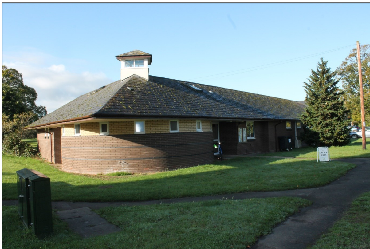
Plate 23: Northern elevation of Parish Hall
