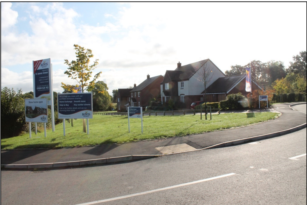
Plate 6: Pippin Drive frontage to Drake Street (part of Lawn Farm Phase 1 development)
