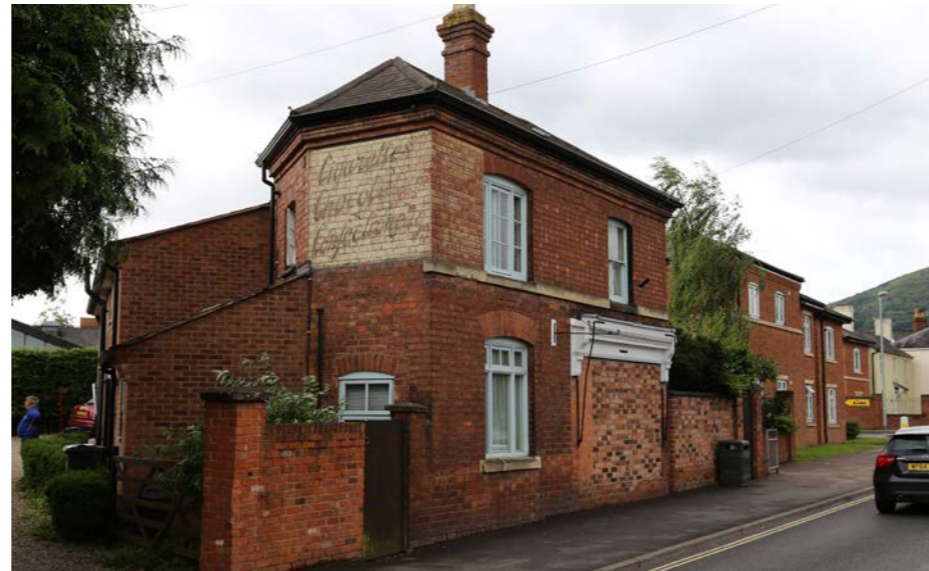
Converted property, Worcester Road
