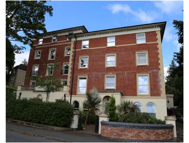
21st century apartment building
