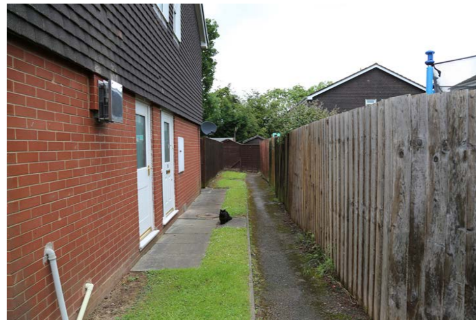
Footway through the character area
