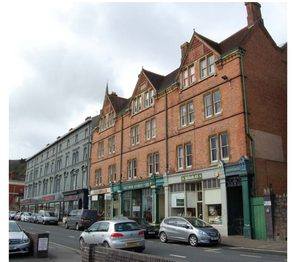
Shop fronts, Worcester Road
