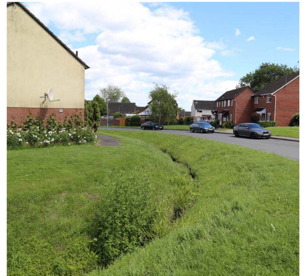
Swale within Harbinger Avenue
