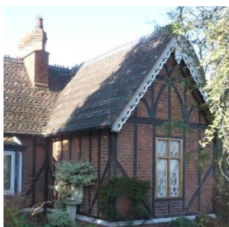
(Bargeboards and decorative roof and ridge tiles)
