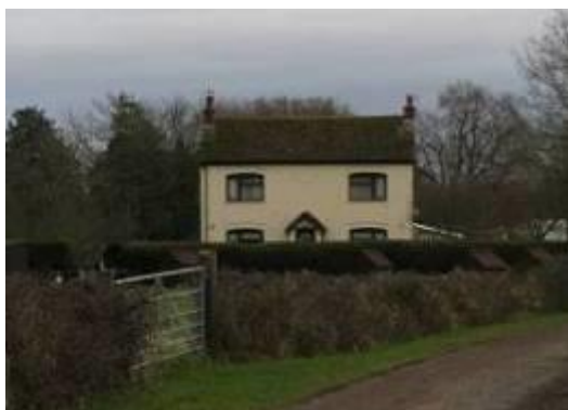
(New windows retain scale and proportions of traditional wayside cottage)
