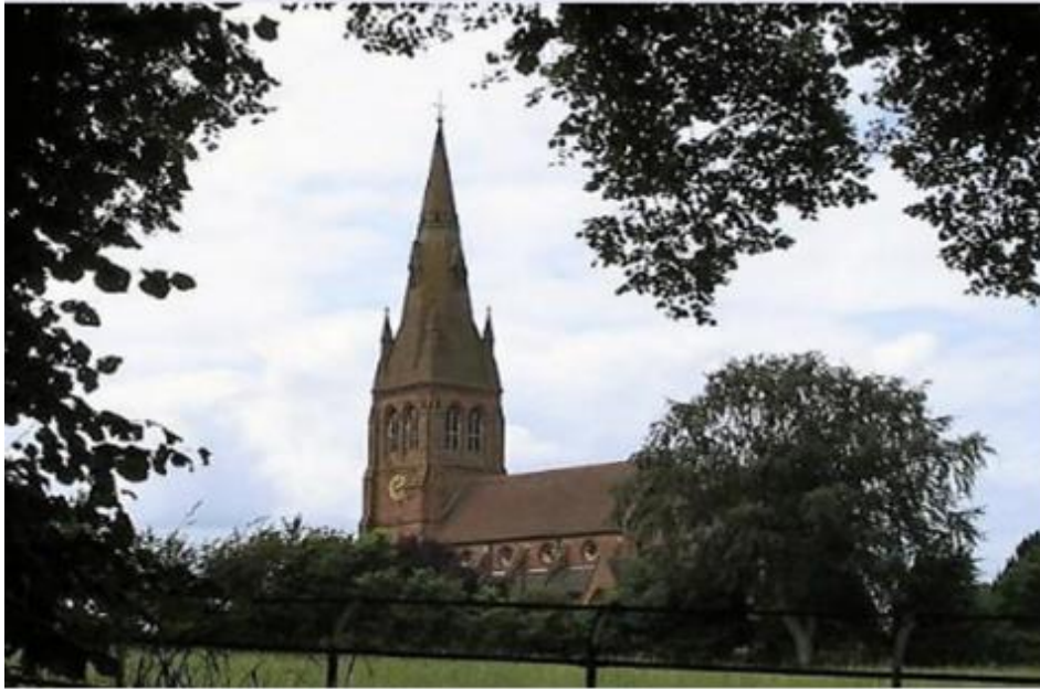
View of Hallow Church from the South
