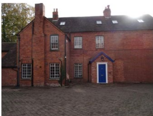
Front elevation facing north, away from Church Lane
